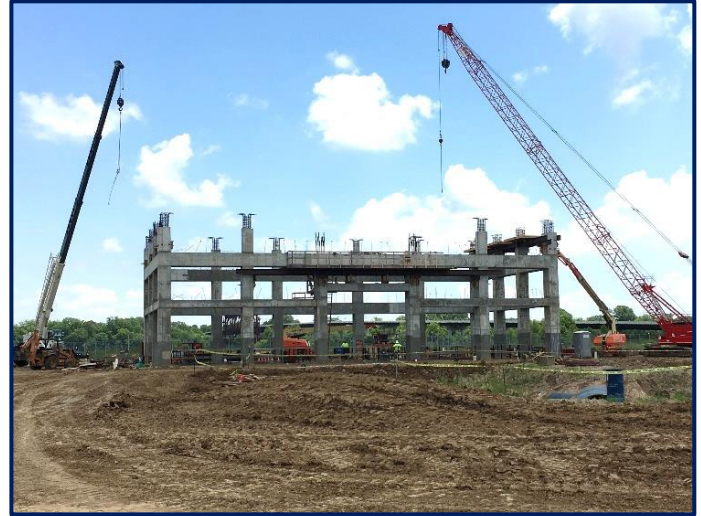
Grand Prairie Pump Station Superstructure, AR.
